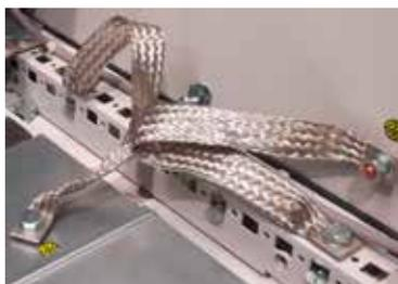
Bonding conductor to manage interference currents generated by the drive
